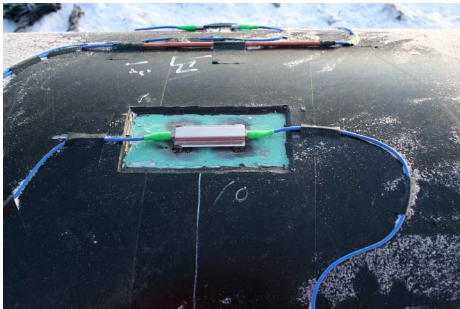
Figure 5. Strain Monitoring Sensors Install on Site in Winter Time
