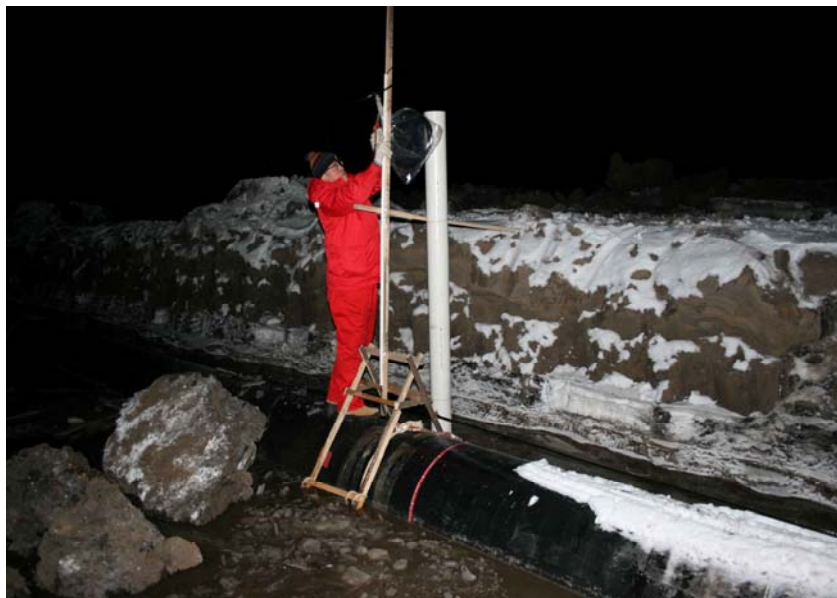
Figure 3. Technical Worker Install Temperature Sensors on Site In Winter Time
