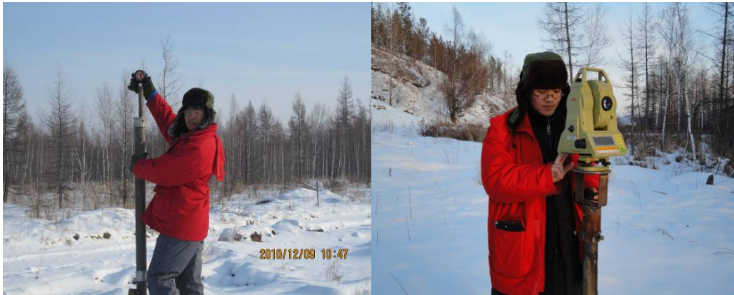
Figure 7. Technical Worker Use Theodolite to collect data on Site in Winter Time
